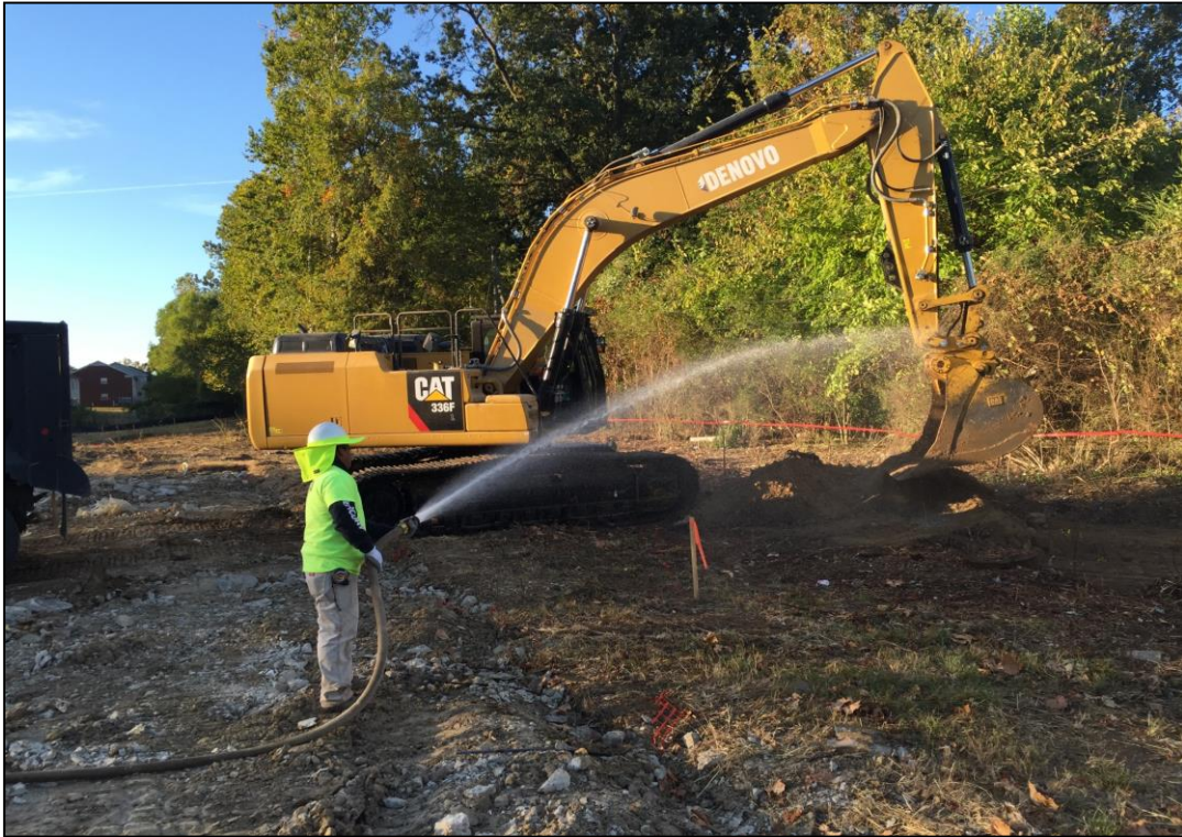
Photograph #10 10/20/15 Photo of dust control during hot-spot excavation.
