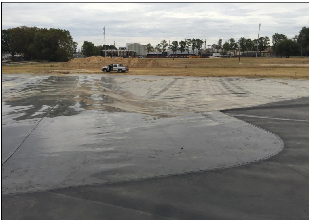
Photograph #13 10/23/16 Photo of Consolidation Area after covering hot-spot soil with HDPE.
