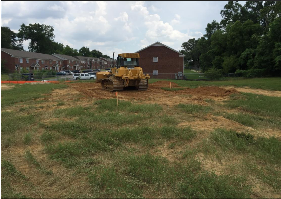
Photograph #24 06/20/16 Photo of cap thickness modifications.
