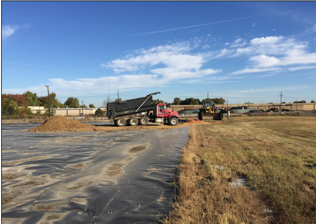
Photograph #12 10/20/16 Photo of hot-spot soil placement at Velsicol Chemical Corporation.
